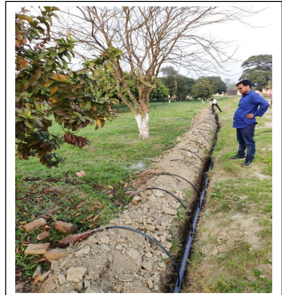
Drip irrigation being laid in orchard
